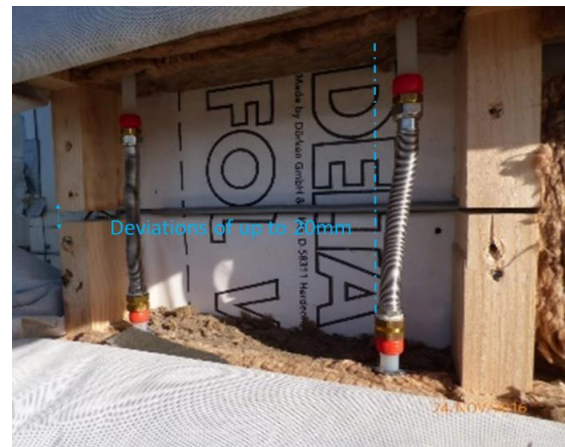
Figure 1: Top: deviations due to assembly inaccuracies. Bottom: deviations during installation.
