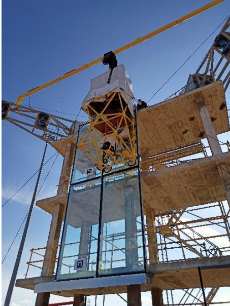
Figure 4: Robotic Installation of Modules with a CDPR.
